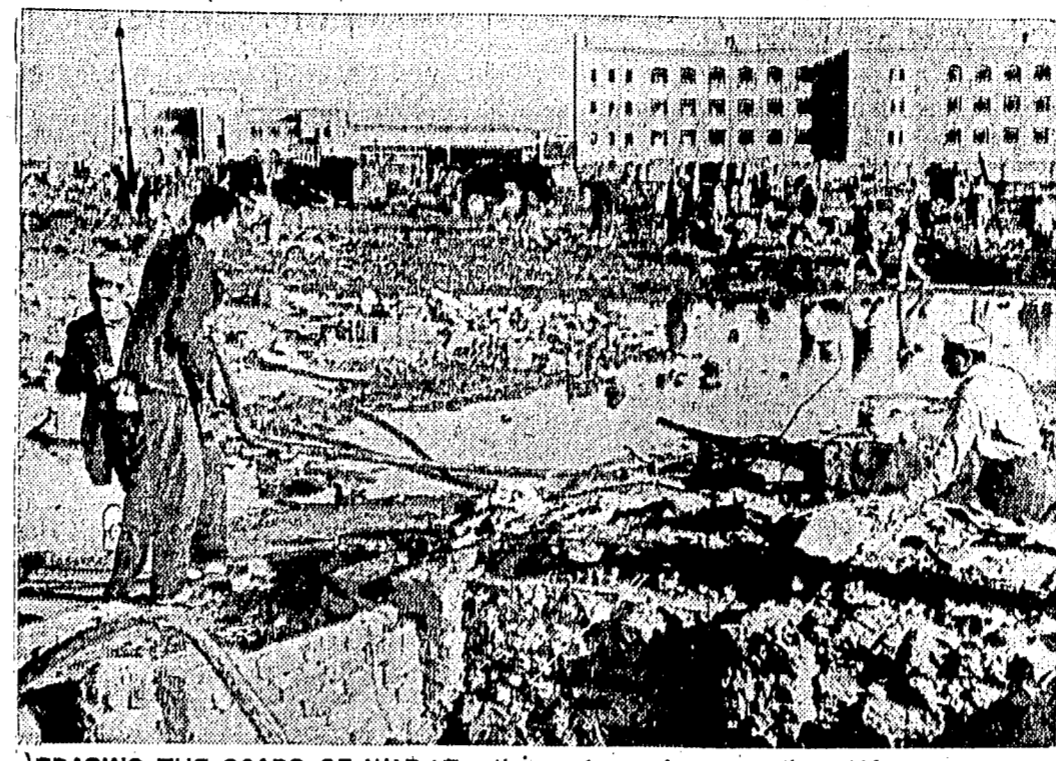
ERASING THE SCARS OF WAR —Egyptian workmen clear away the rubble of buildings smashed by the air and sea bombardment which accompanied the Anglo-French invasion of Port Said. The United Nations salvage fleet has resumed efforts to clear the blocked Suez Canal, of which Port Said is the northern terminus.
