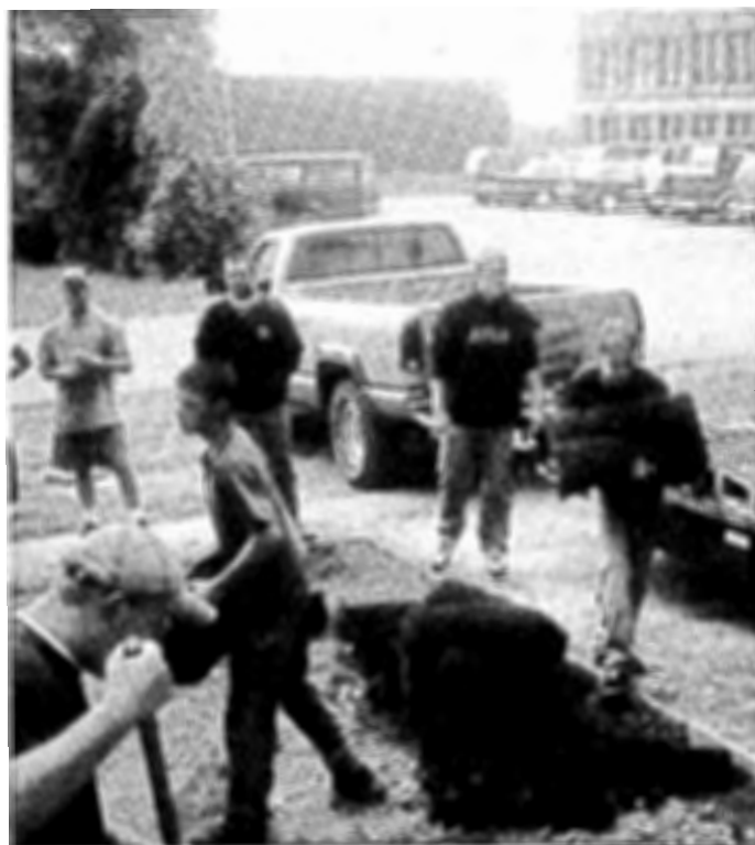
It's a dirty job, but someone has to do it. The building construction class helps put the finishing touches on the Habitat for Humanity house the class helped construct.
